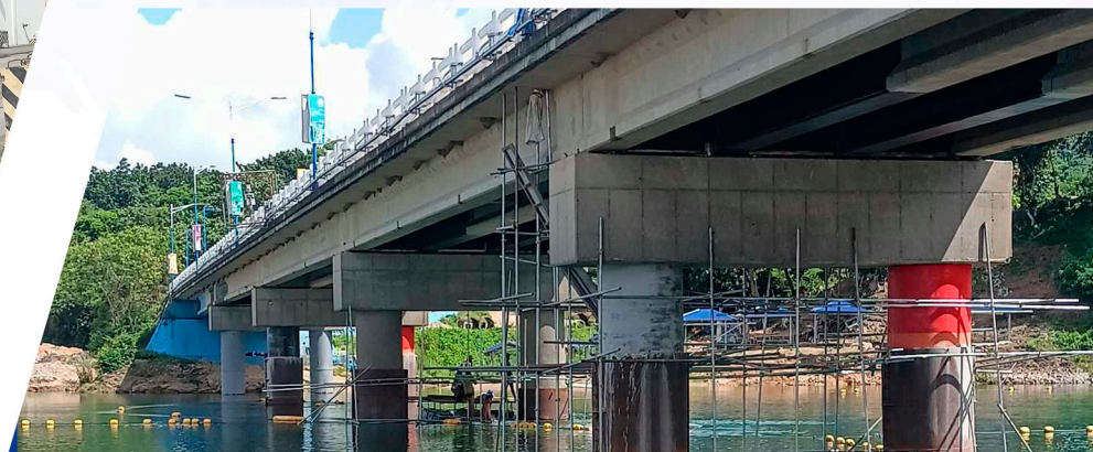
Ilagan-Bigao-Palanan Road, Ilagan, Isabela, Cagayan Valley Products used: Solidcure
