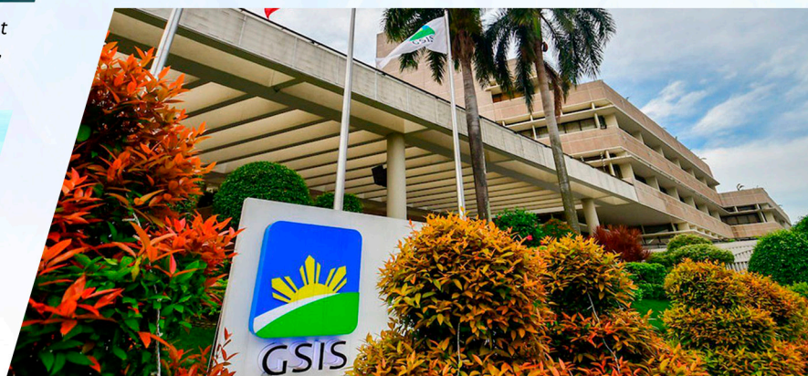
GSIS Building Products used: Epocoat MB Primer, Blockout Hyperblock Aqua, Floortek Shield, Blockout 40 Strip, Handy Fix Pro
