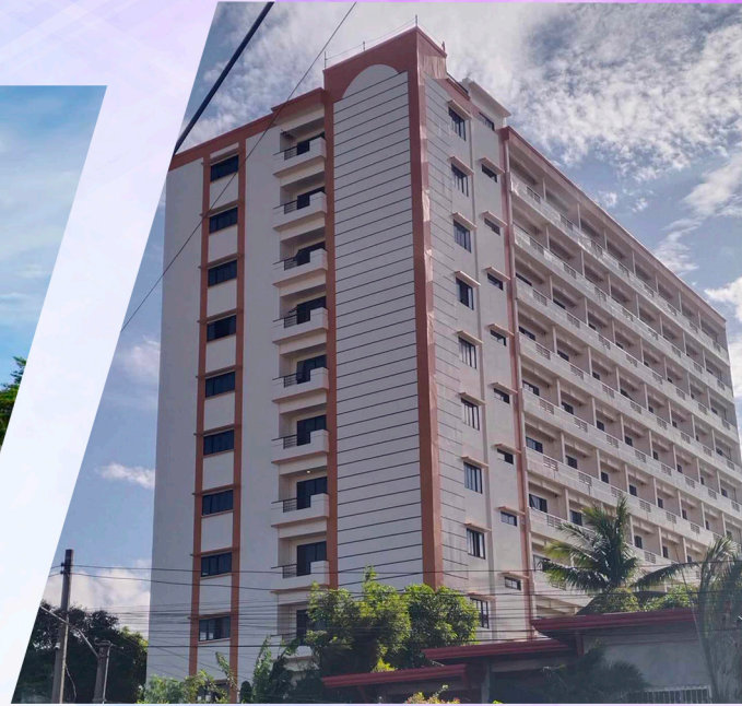
August Residence Tabucan, Manduriao Iloilo City Product used: Waterroofing-Crystor, Leakplug, Epocoat MB, Blockout ETL, Cementgrip, Confix IJ, HV, Sapal RTU
