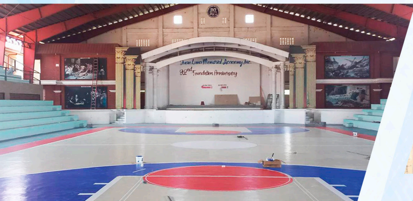
Marcos Sports and Cultural Building, Sisa, Manila
