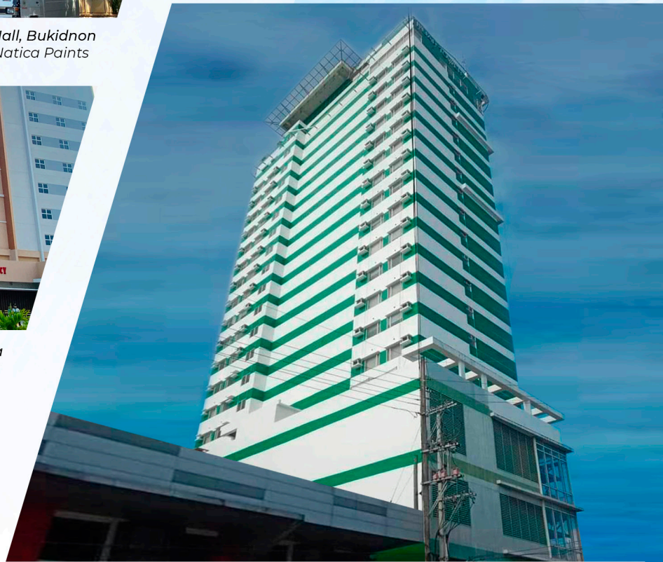
INJAP Tower, Manduriao, Iloilo City Products used: Sapal 2-in-1, Confix IJ, Stoppag FS, Stoppag 1, Sinclair Natica Paints
