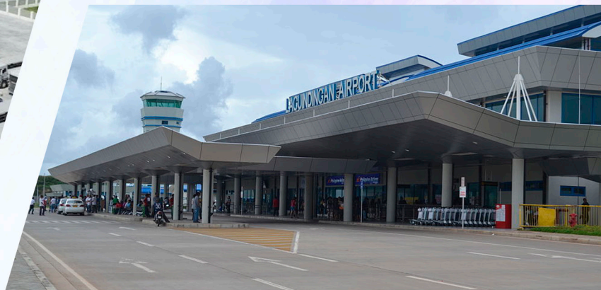
Laguindingan Airport, Habini Bay, Misamis Oriental Products used: Confix IJ, Confix HV, Leak Plug, Handyfix, Epocoat MB & Cleversil
